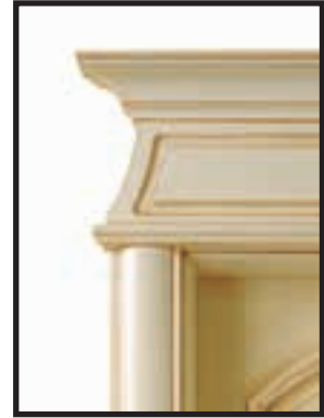
Trim Detail Paint Grade Poplar Julia Casing CS402DL & Custom MDF Header
